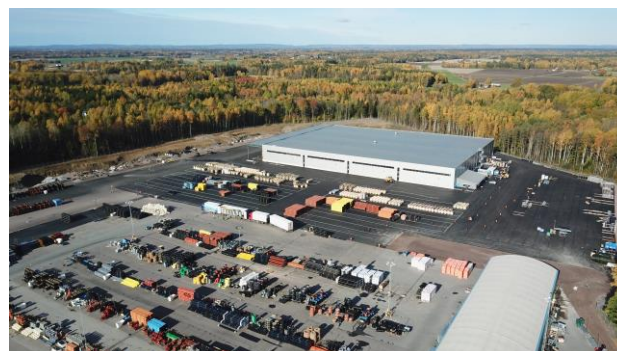
The new pipe warehouse at the Swedish central warehouse was inaugurated in October.
