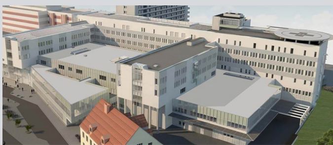
Eskilstuna Hospital construction site
